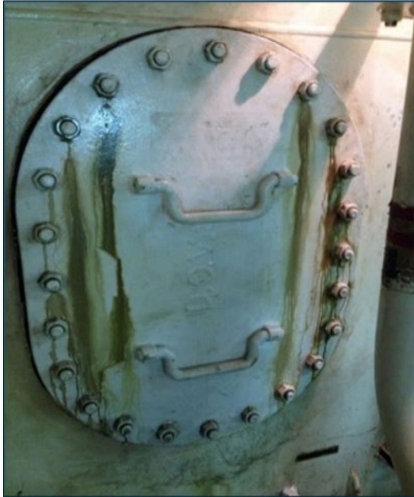
Leaking manhole cover (diesel oil tank).
