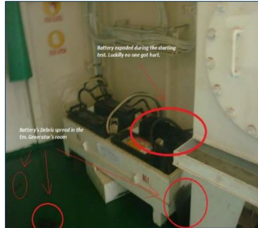
Emergency generator batteries explosion during testing
