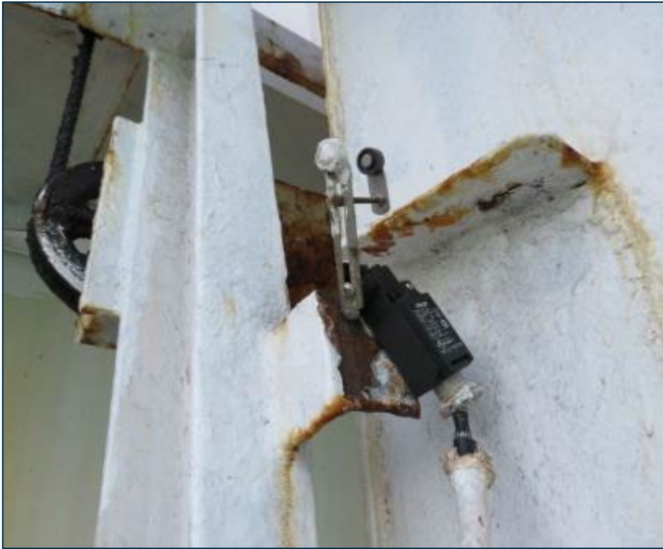
Defective / seized limit switches
