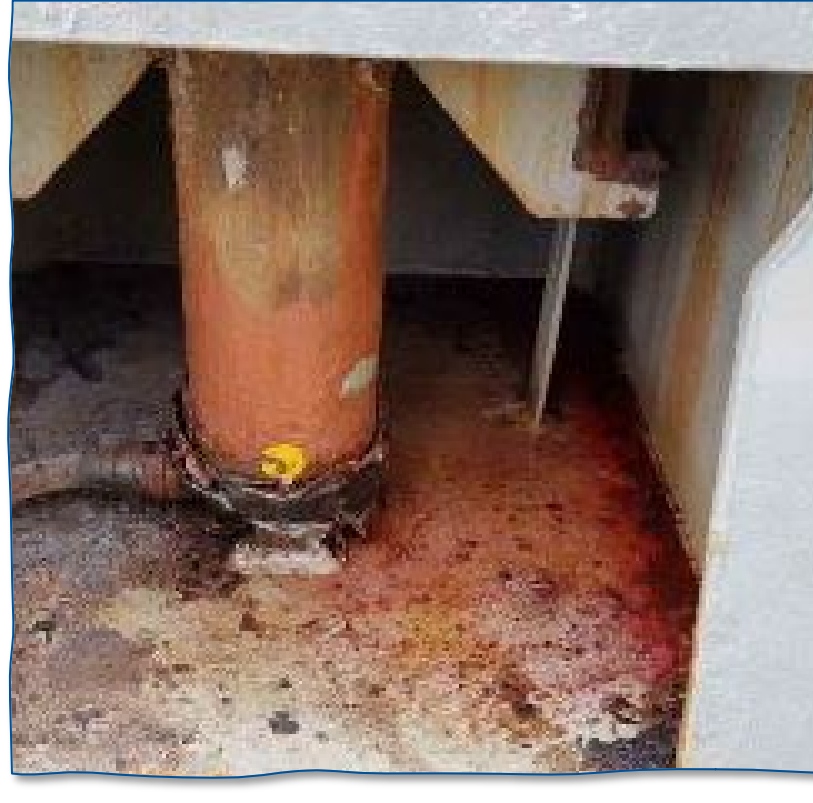
Hydraulic leaks
