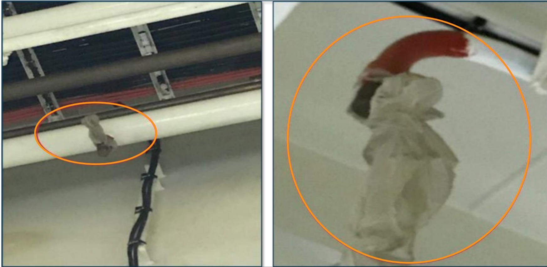
Hypermist nozzles wrapped in plastic
