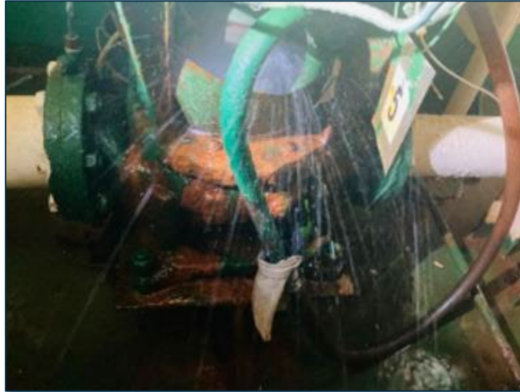
Leaking EFP gland packing / mechanical seal
