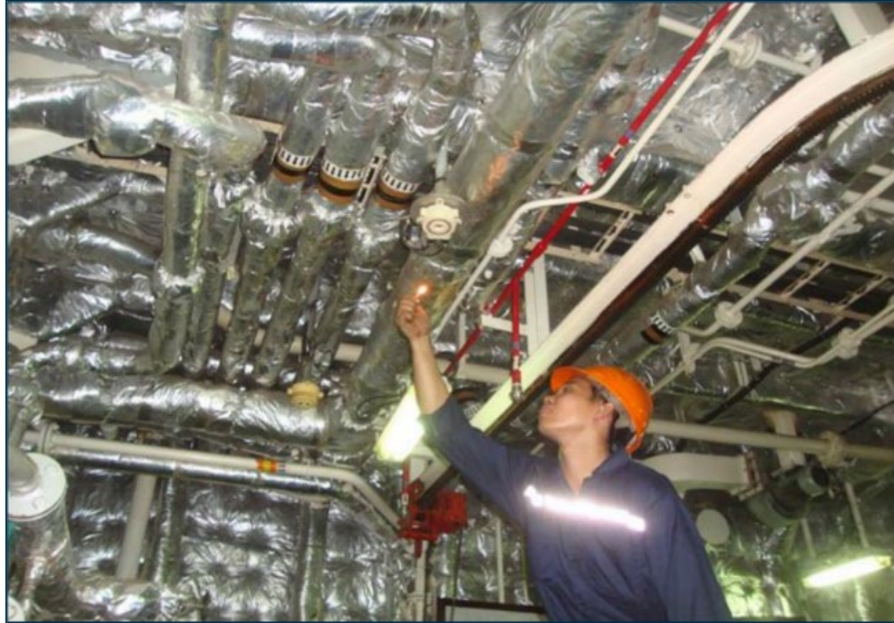
Heat detector inappropriate testing material
